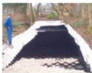
Installation of the CellWeb™ system.
