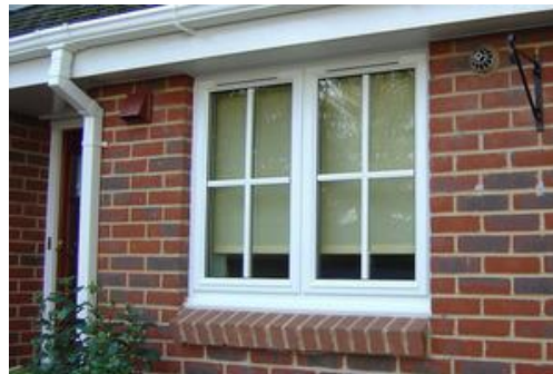
Aluminium casement window with powder coated white finish
