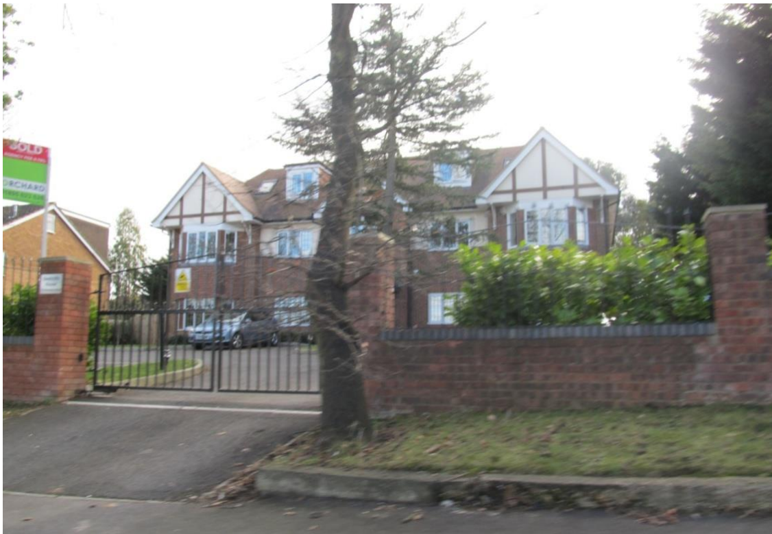
Development of 8 flats at 179 Swakeleys Road
