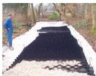
Installation of the CellWeb™ system.
