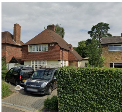
Images 3.1.2f and 3.1.2g above show 20 Kingsend and 40 Kingsend with vertically hung tiles
