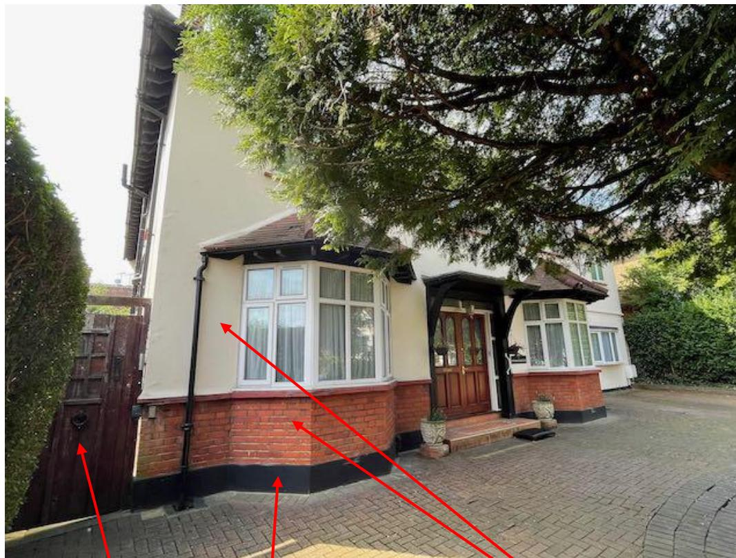
Existing wooden side gate and frame to be adjusted for thickness of external wall insulation and re-installed.
