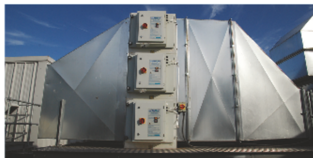
3 ESP Units Stacked in modular formation
