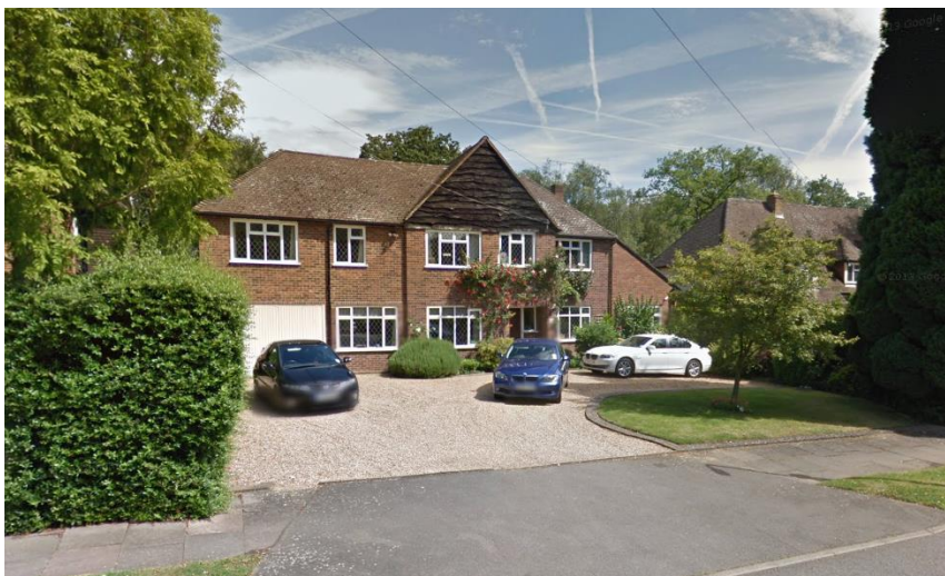
2. View from Street (towards neighbours dwelling No. 97)
