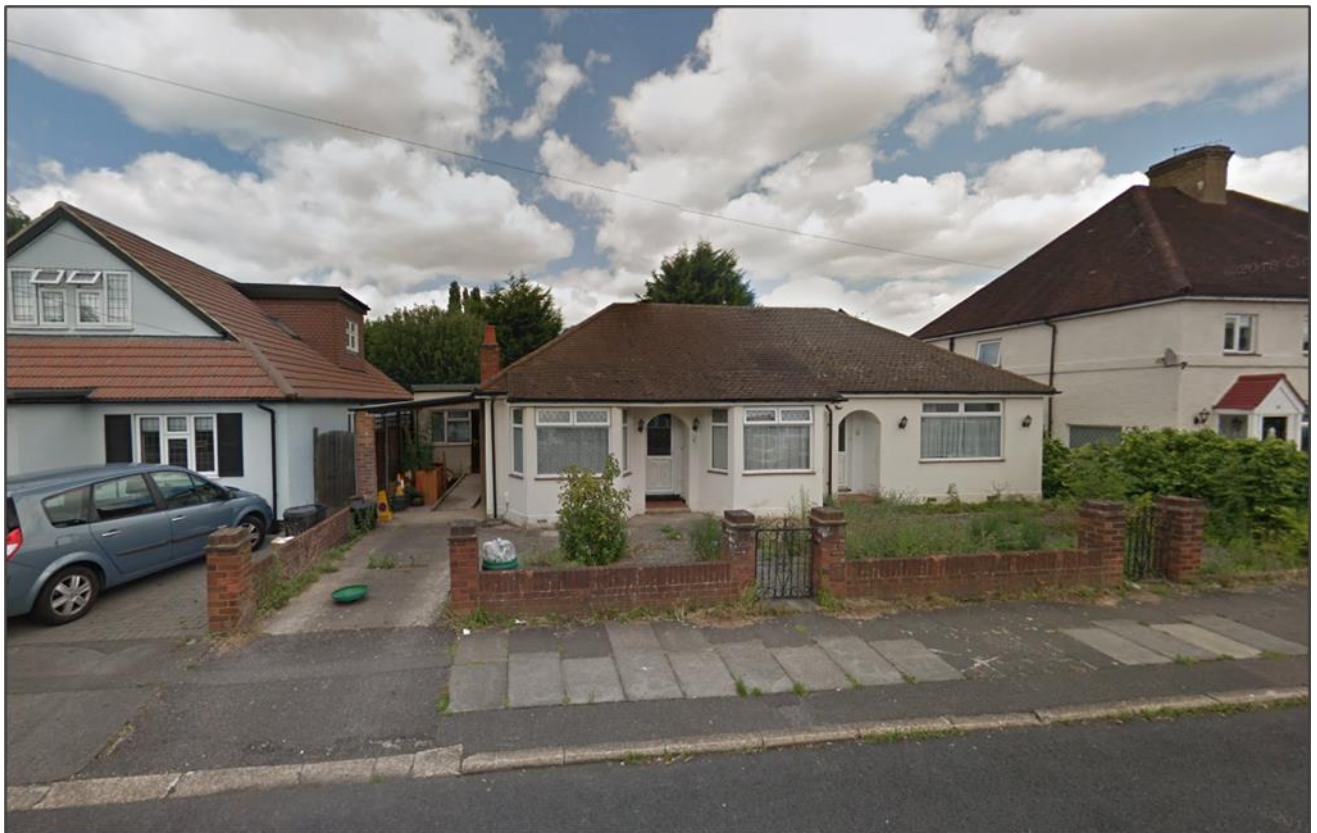
Figure 1 – The Application Site
