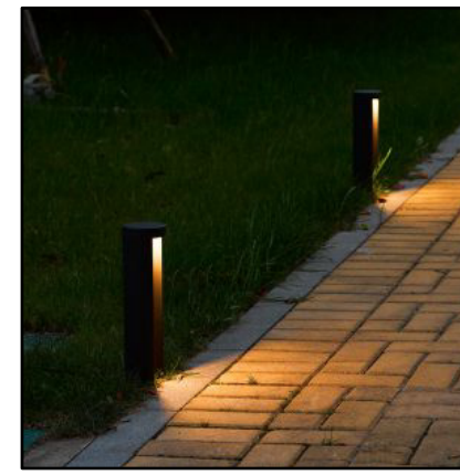
Bollards lighting driveway
