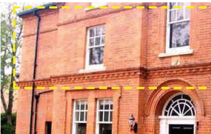
Picture 1, Red brick banding details and visual example (read with drawing A-42)
