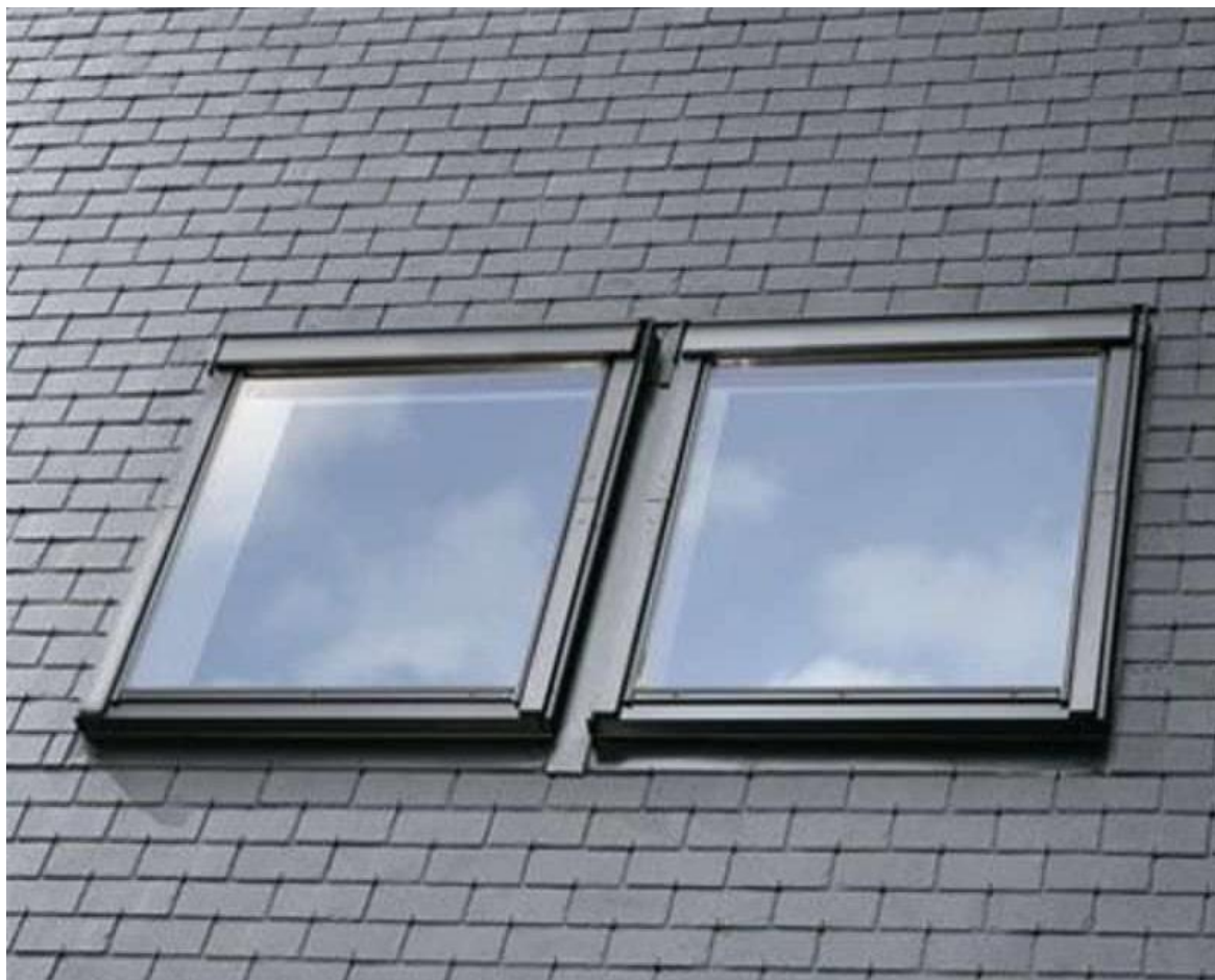
Picture 7, Grey slate tile roof and Timber Skylights
