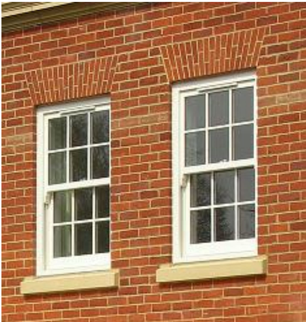
Picture 3, Windows visual example. Red brick soldier course above the sash windows and sills
