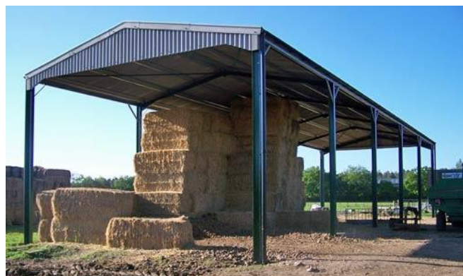
Figure 3 - Indicative Appearance of Barn 1
