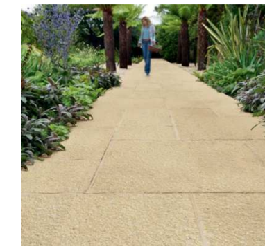
2 600x600 PAVING SLABS TO REAR PATIOS AND FOOTPATHS, IN NATURAL COLOUR.
