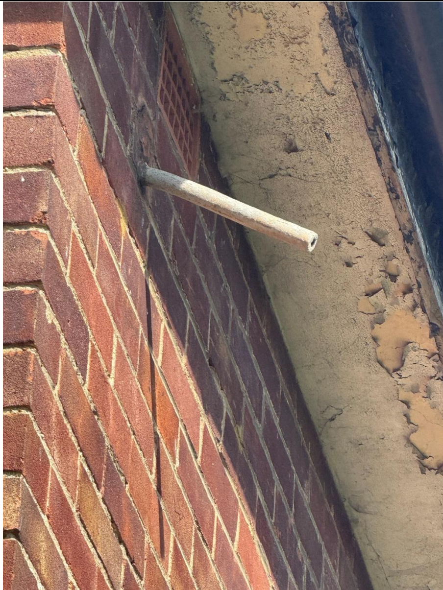
Close fitting soffit
