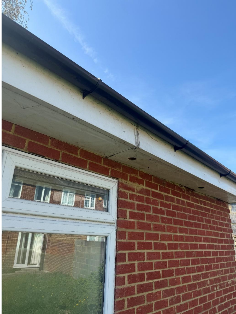
Soffits showing access holes
