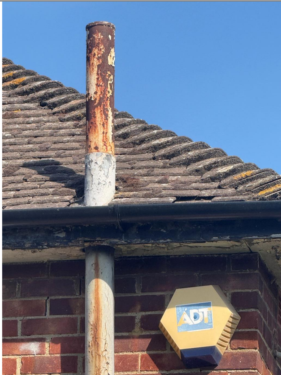
Gap under roof tile at rear of building
