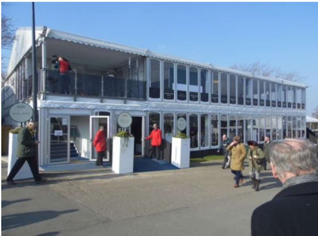
Similar structure (for reference)
