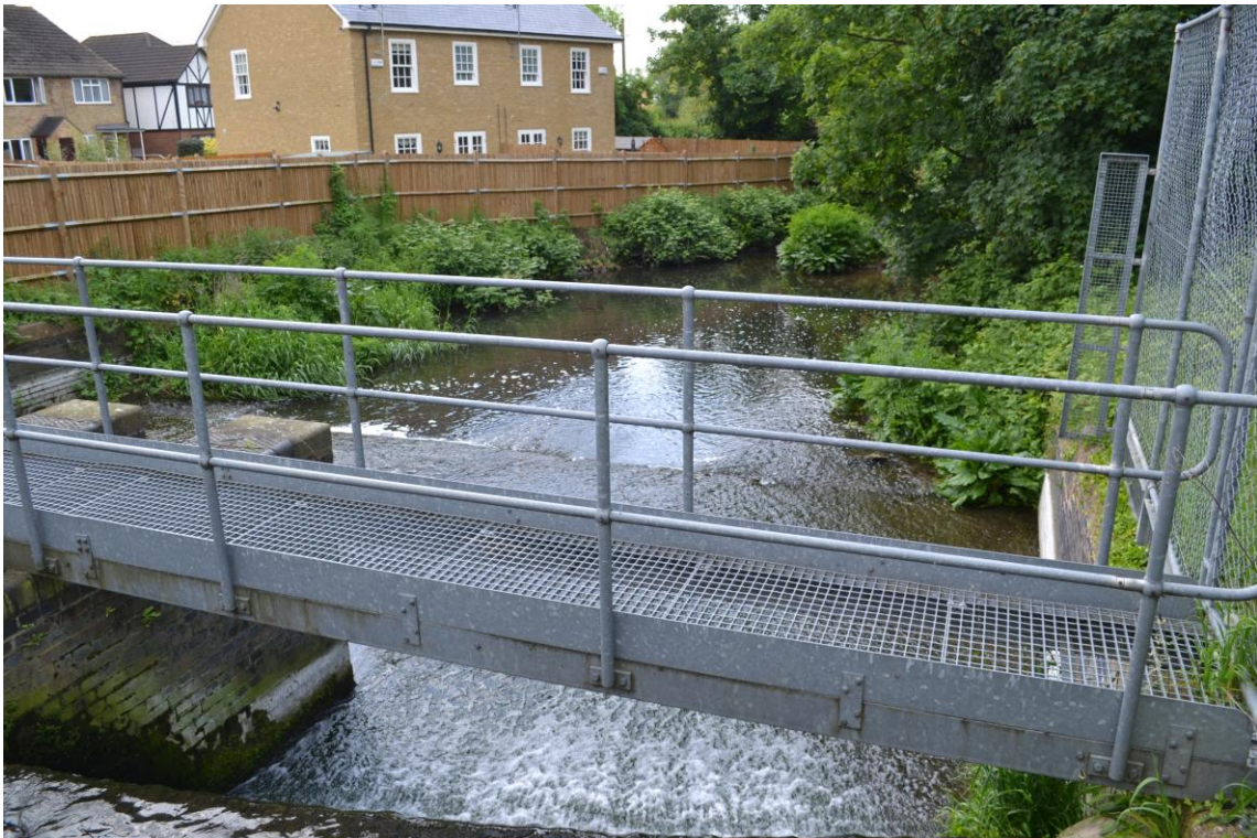
Lateral weir from Grand Union Canal to The Culvert looking west
