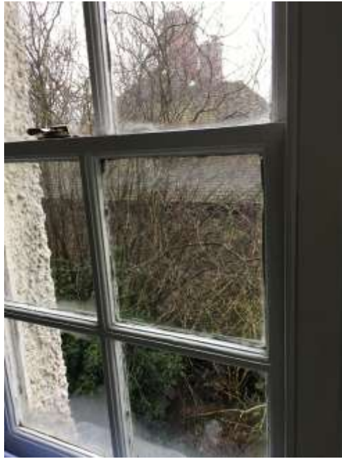
Photograph 5 - First floor side window to Sadie's bedroom
