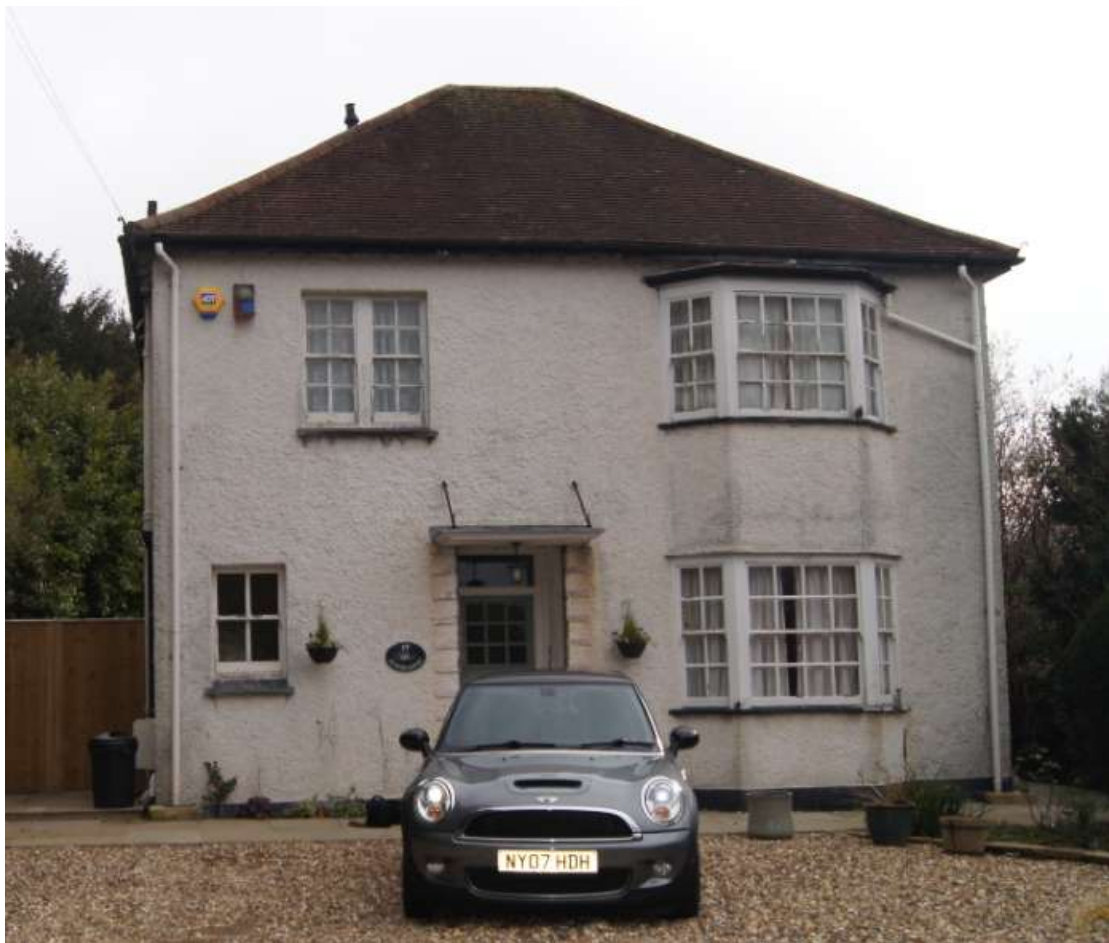
Photograph 4 - Front facade of 17 Elgood Avenue
