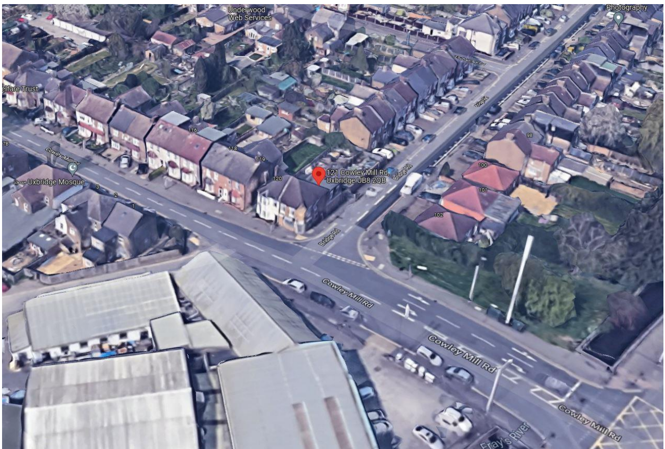
Fig 3. Aerial view of site from south west.
