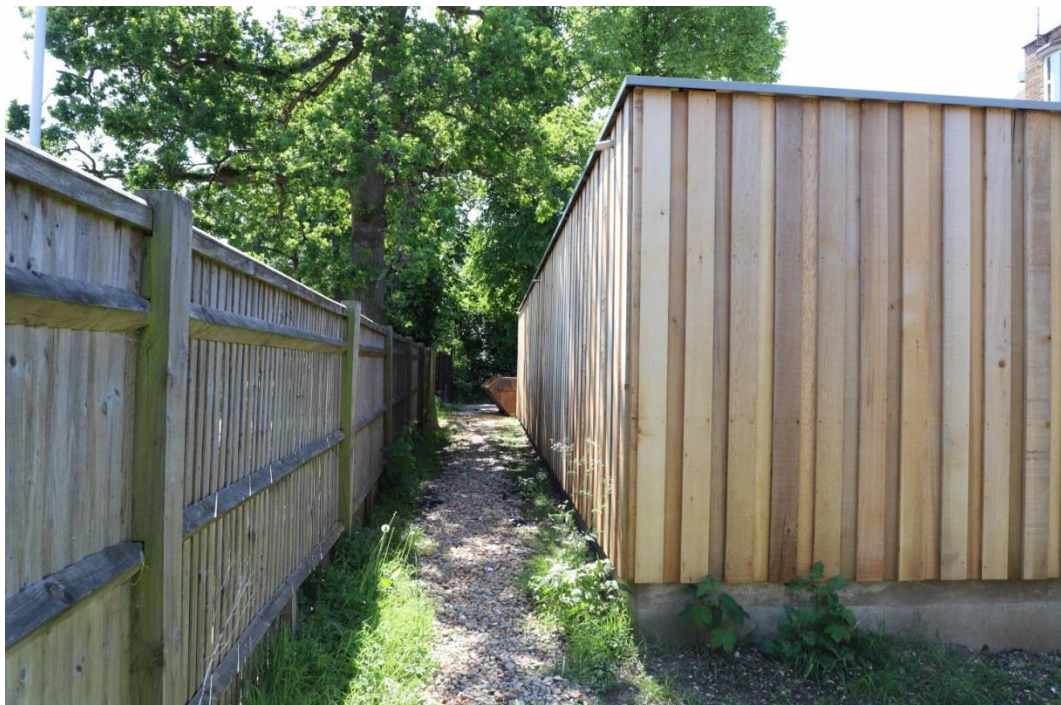
View of passage between boundary fence and store. This will be planted with Photinia red robin for the entire length. Planted height to be 1500 to 2000mm with future growth 3500mm high which will mask the store from the road
