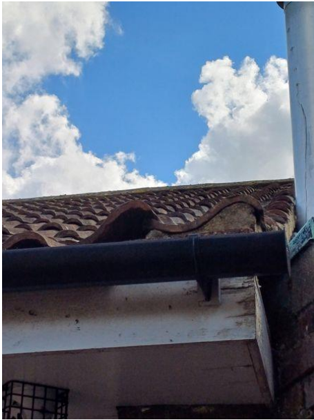
Plate 4.9: Gap due to missing mortar under end tile on western elevation
