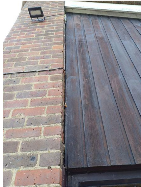
Plate 4.10: Gap between weatherboarding and external wall on northern elevation
