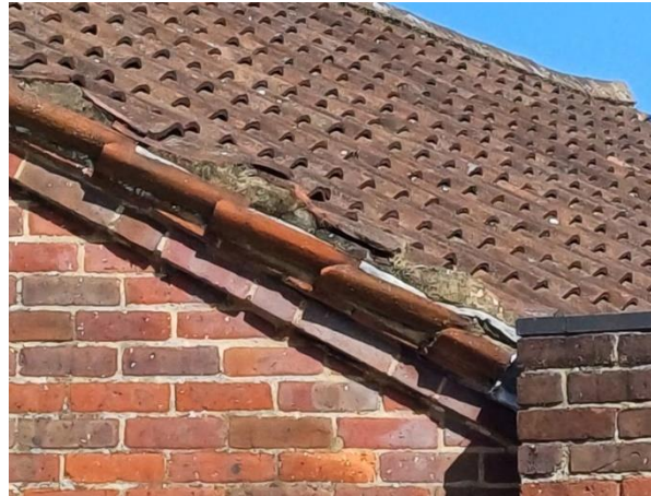
Plate 4.6: Missing mortar under roof tiles on southern elevation
