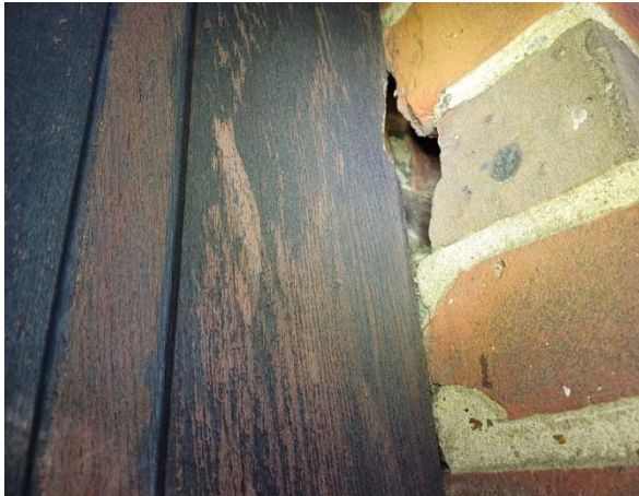
Plate 4.5: Gap between weatherboarding and external wall extending into cavity on southern elevation
