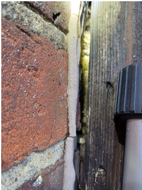
Plate 4.3: Gap between weatherboarding and external wall on southern elevation
