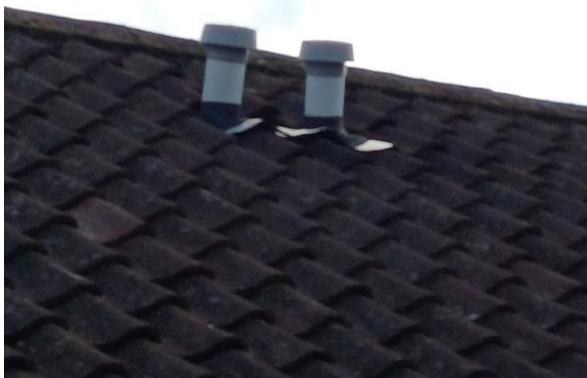
Plate 4.11: Lifted lead flashing around central chimneys
