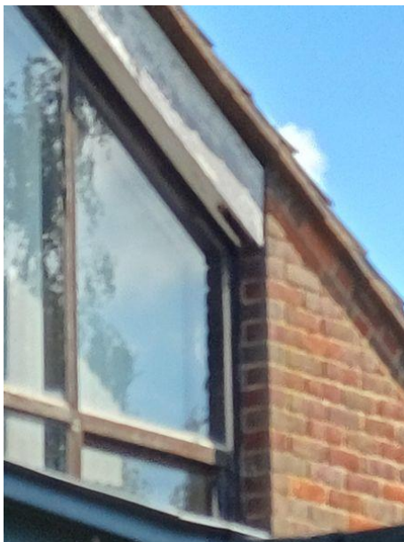
Plate 4.7: Gap caused in fascia board by wood rot on southern elevation
