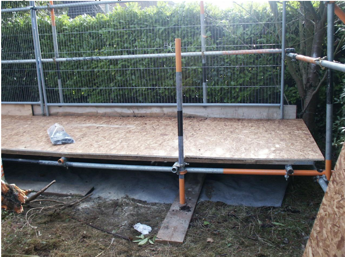
Photo 3 Scaffold framework supporting wooden boards
