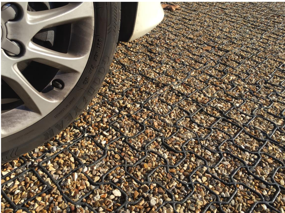
Photo. An example of a finished Gravel Grid system
