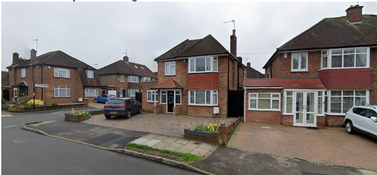
Figure 1- Street view from Hoylake Cres which shows the existing ridge level is lower than the adjacent buildings
