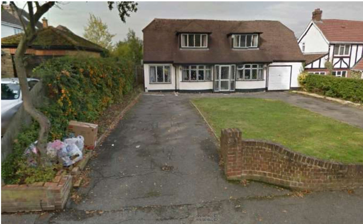
Existing house that is proposed to be demolished
