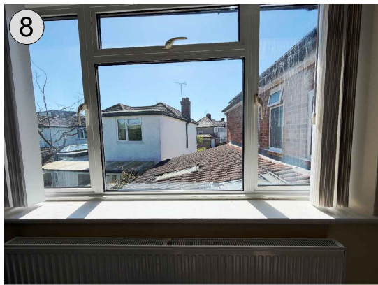
First Floor Room Window Towards Front 1
