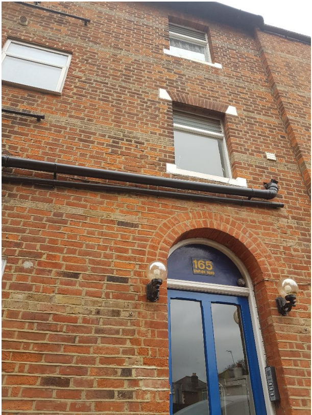
View of west showing entrance into building (common parts)
