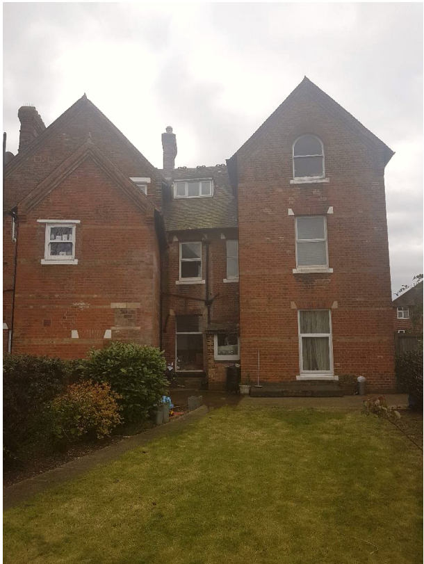
View looking south west (rear) of application site
