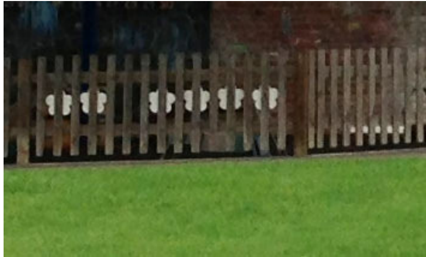
Figure 2. Existing timber palisade fence
