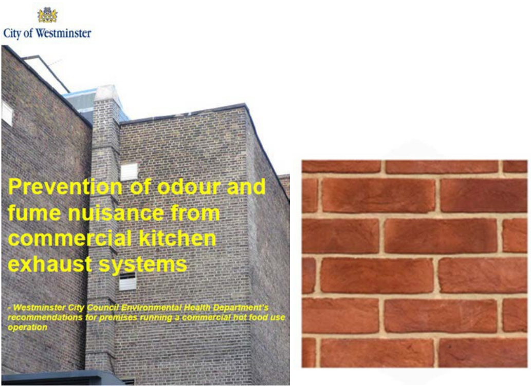
Example of an extract design concealing the flu in matching finish to the host building. The Sample Red brick is the proposed finish type of wrap we proposed to install around the visible elements of the vertically flu.
