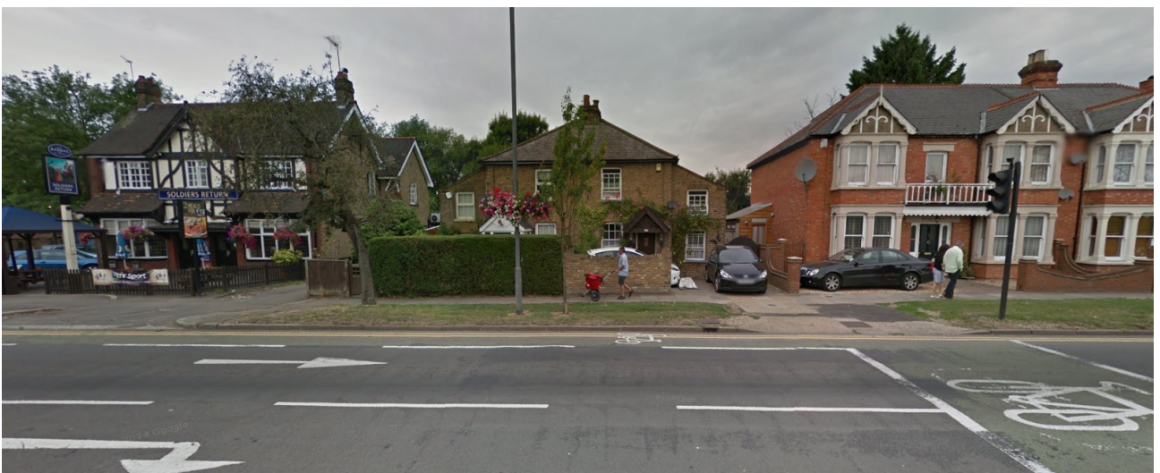
Photo 03 View from the main elevation. The proposed extension will be sympathetic to the area and surrounding buildings
