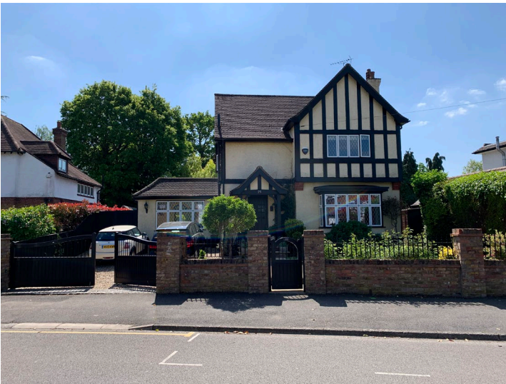
25 Manor Road Street Elevation
