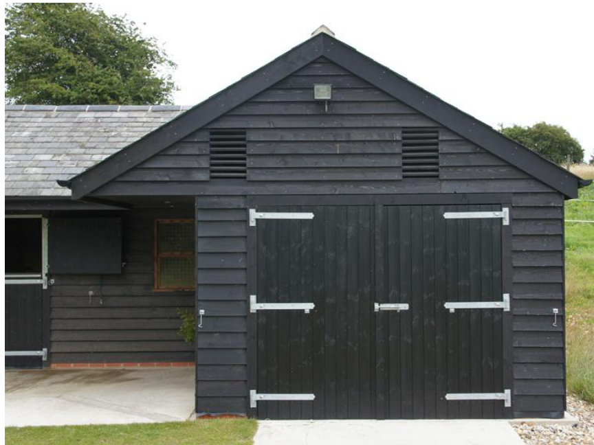
Image example of stable door
