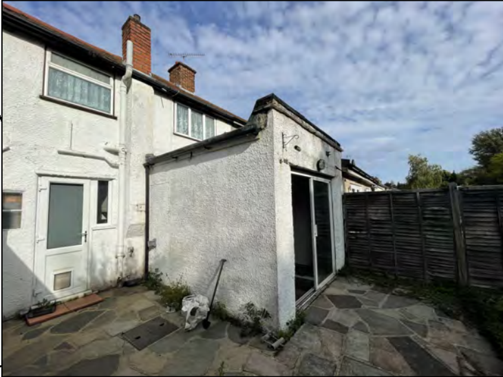
EXISTING REAR HOUSE ELEVATION SITE PICTURE
