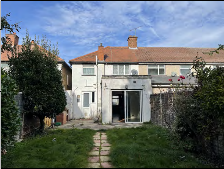
EXISTING REAR HOUSE ELEVATION SITE PICTURE
