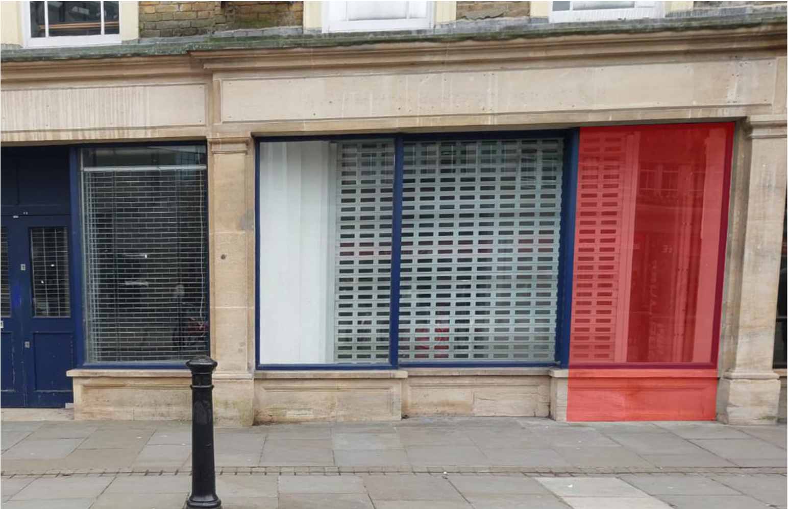
The image above (taken 22/03/2023) shows the area of the existing glazing and stone plinth that will be carefully removed to make way for the new entrance way.
