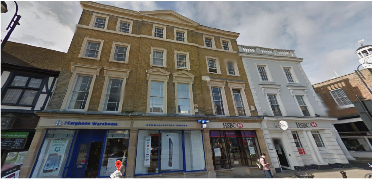
Photo 1- Frontview of 25-26 High Street, Uxbridge-former Carphone Warehouse shop on ground floor
