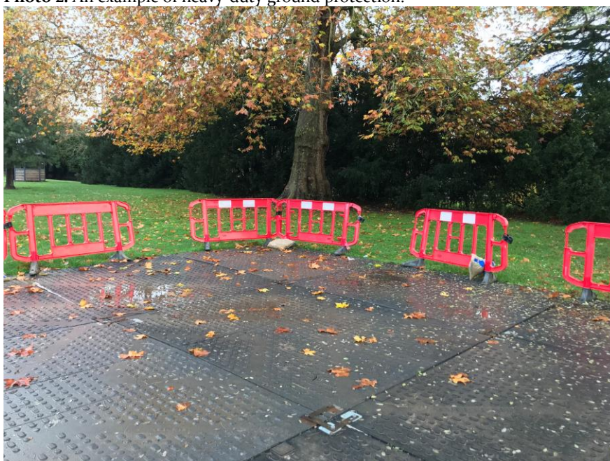
Photo 2. An example of heavy-duty ground protection.
