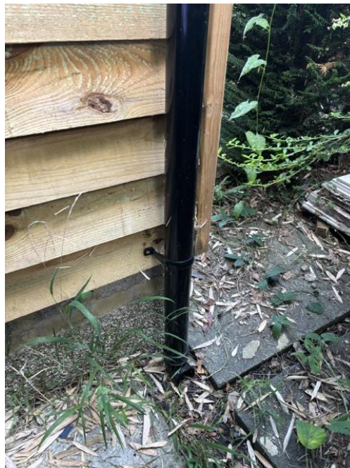
Figure 7. Existing Rainwater Downpipe to Outbuilding
