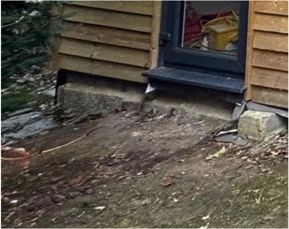
figure 6. Raised base and existing ground level around the outbuilding
