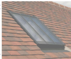
CONSERVATION ROOFLIGHT Suitable for plain roof tiles & to give a seamless flush finish.
