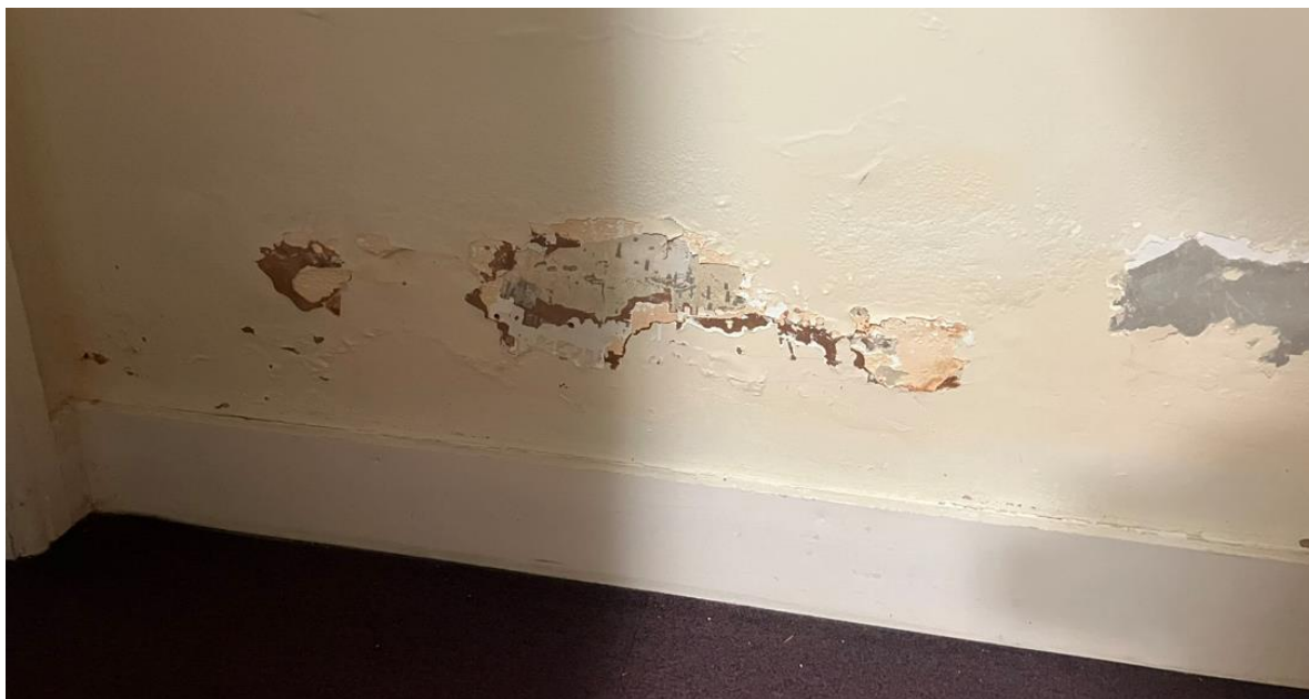
Figure 5 – Water damage to ground floor wall in corridor
