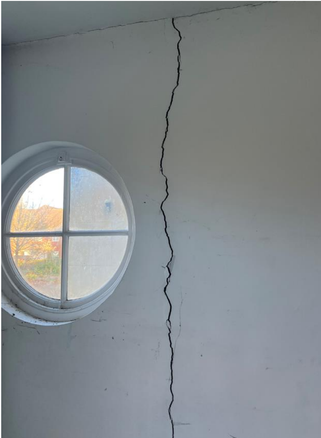
Figure 1 – Crack in wall by round window
