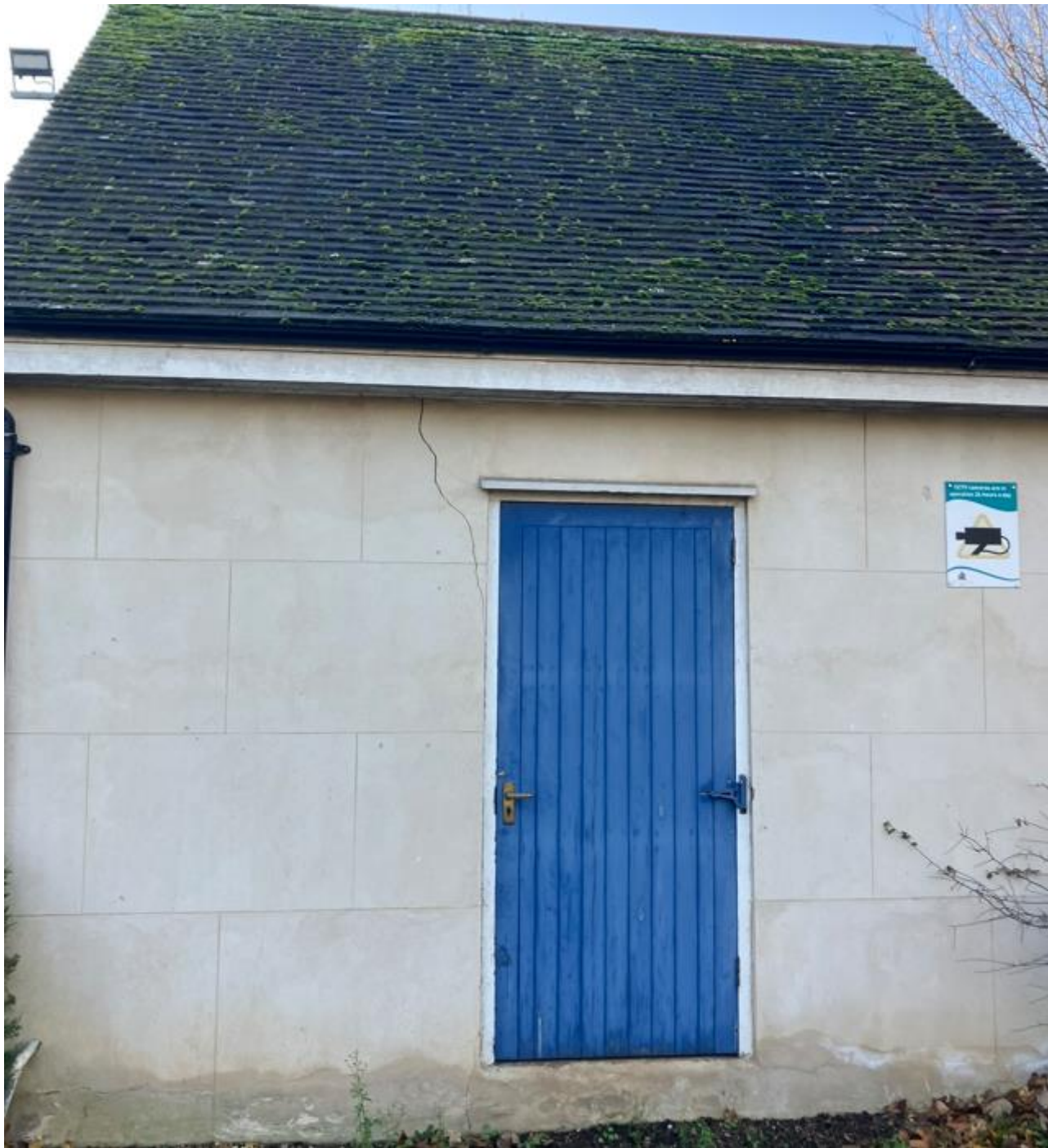
Figure 7 – Crack to wall over doorway in Boiler House
