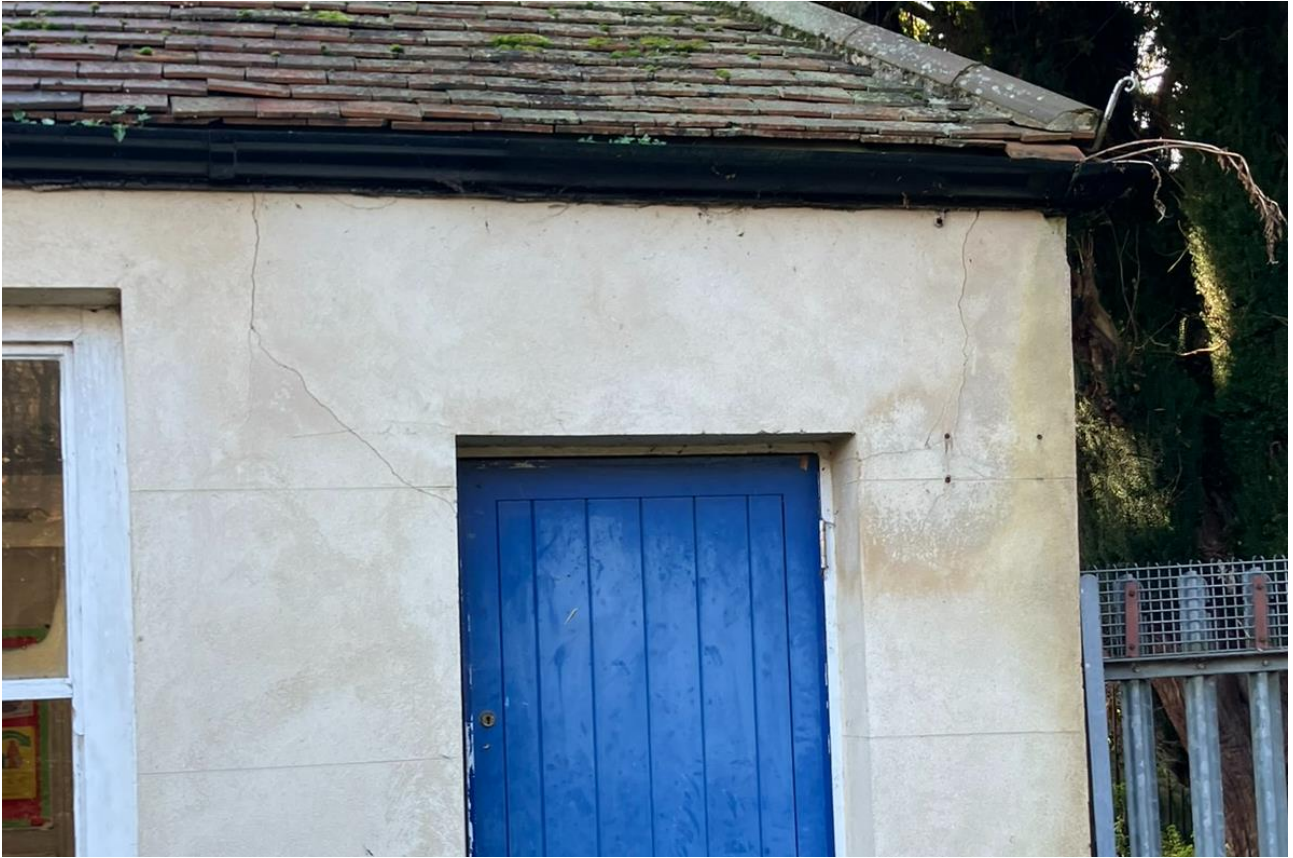
Figure 3 – Cracks to wall over doorway of kitchen
