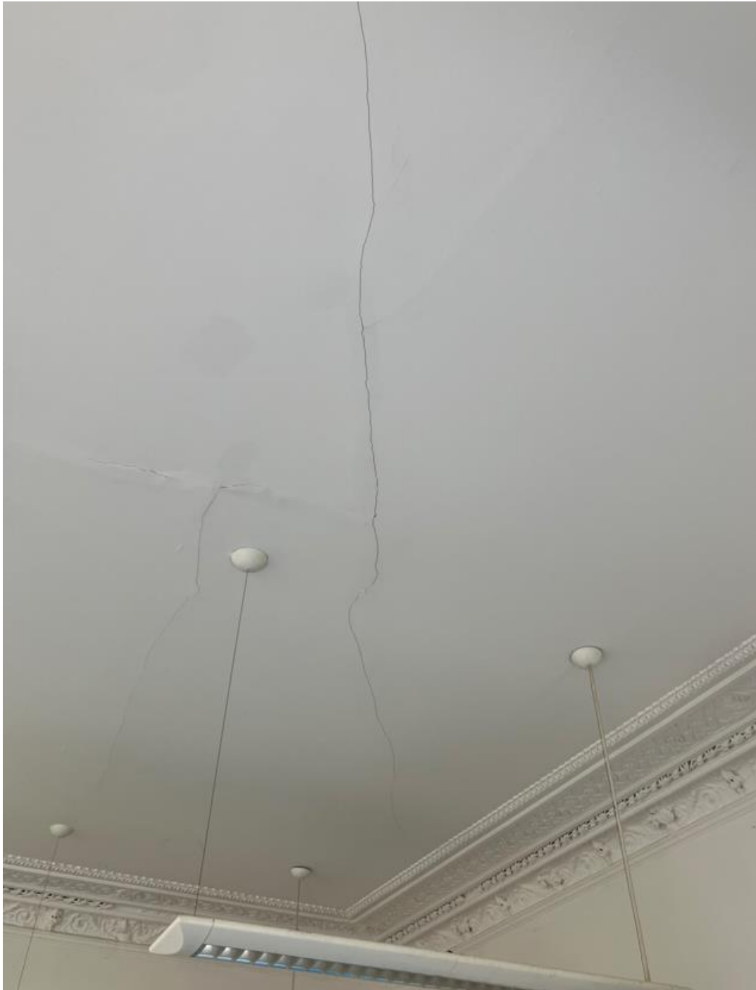
Figure 9 – Ceiling crack over Creche
