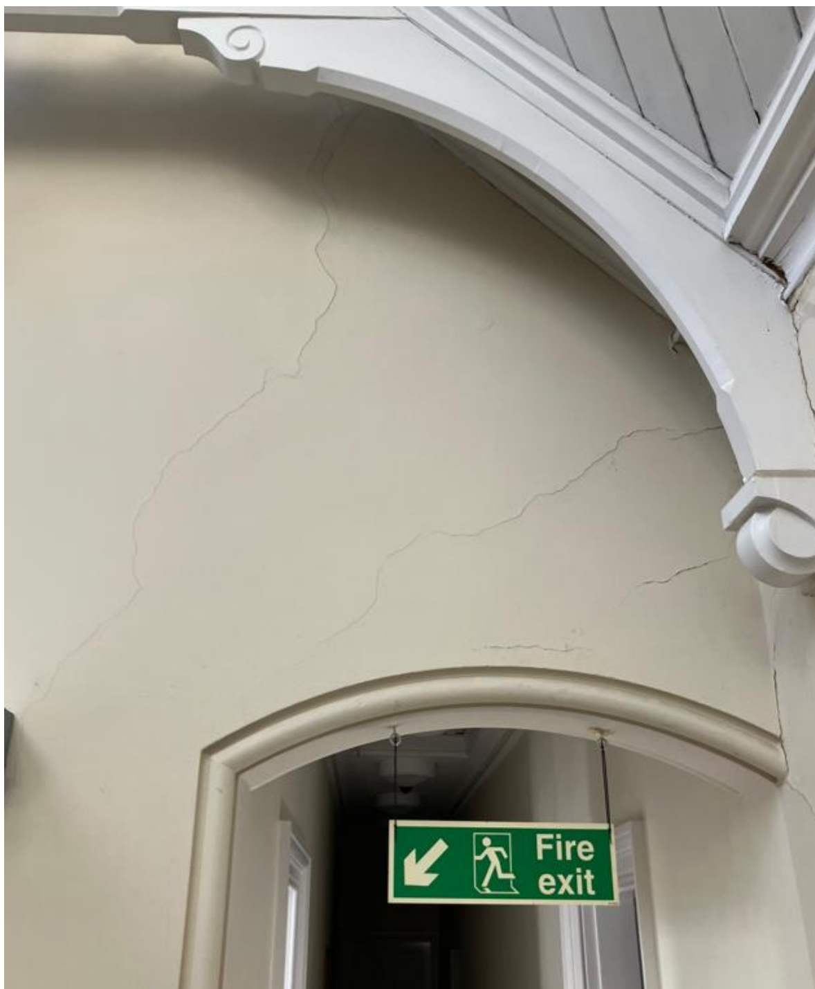
Figure 2 – Crack to wall over landing in hallway
