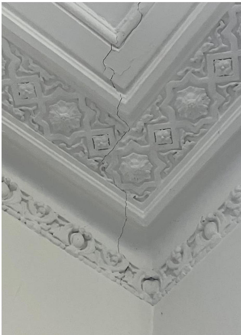
Figure 11 – Typical Cornice damage
