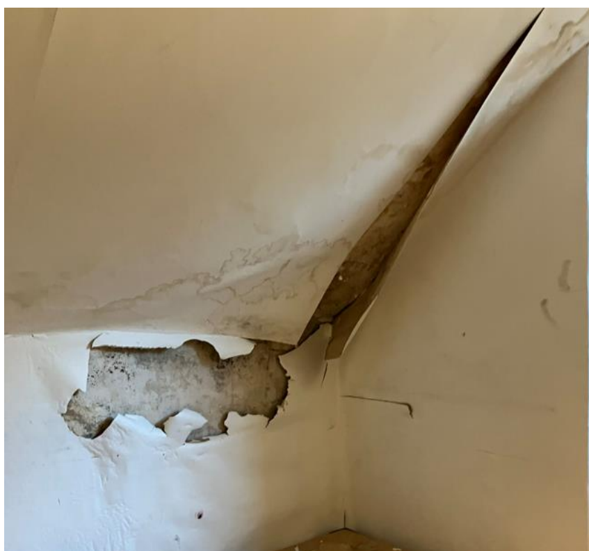
Figure 6 – Water damage to roof structure in first floor meeting room
