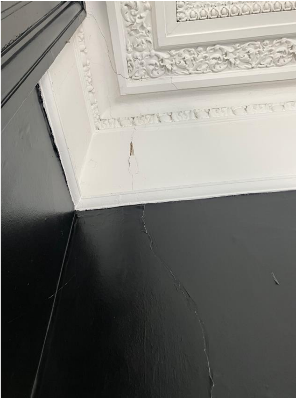
Figure 8 – Vertical wall crack in the Sensory Room
