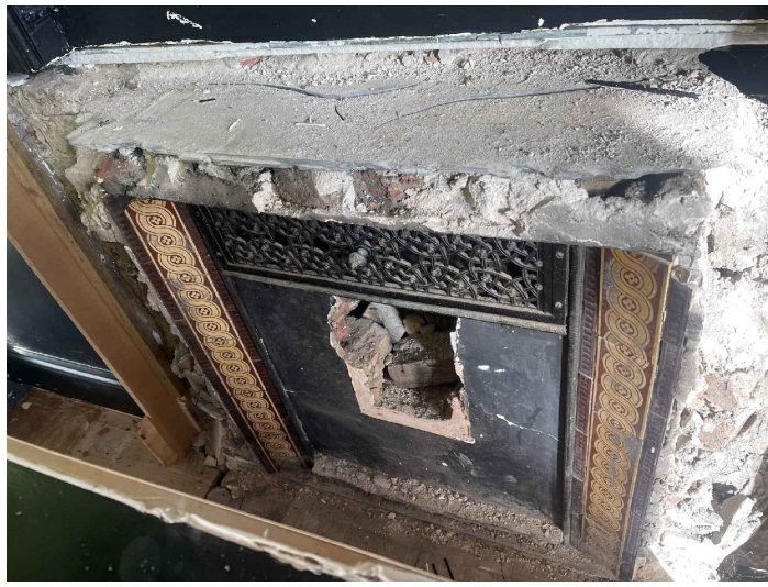
FP2 - Missing mantle and surround. Blocked fire chamber.
