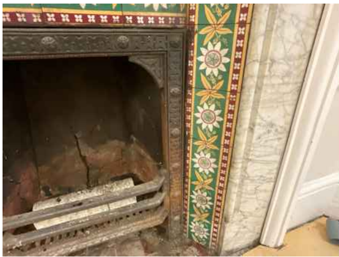
FP4 - Damaged tiles & fire chamber.
