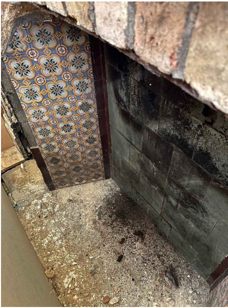
FP1 - Missing mantle & surround. Damaged tiles. Blocked fire chamber.
