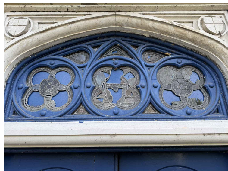
Stained glass damage
