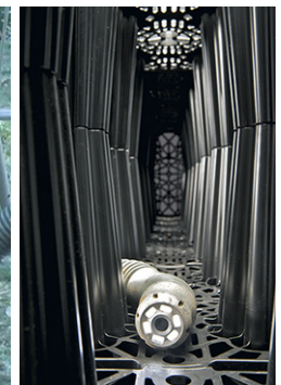
ACO StormBrixx geocellular crates with CCTV inspection cameras inside
