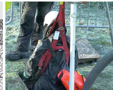
Inspection of ACO StormBrixx HD, geocellular system via a man access unit
