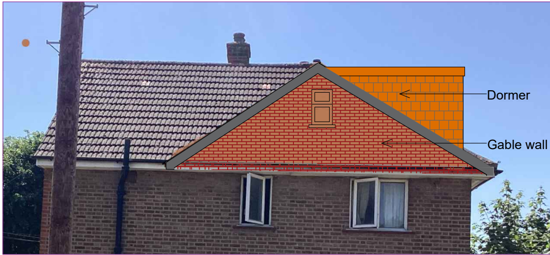
Flank Elevation (RHS) with Gable wall & Dormer
