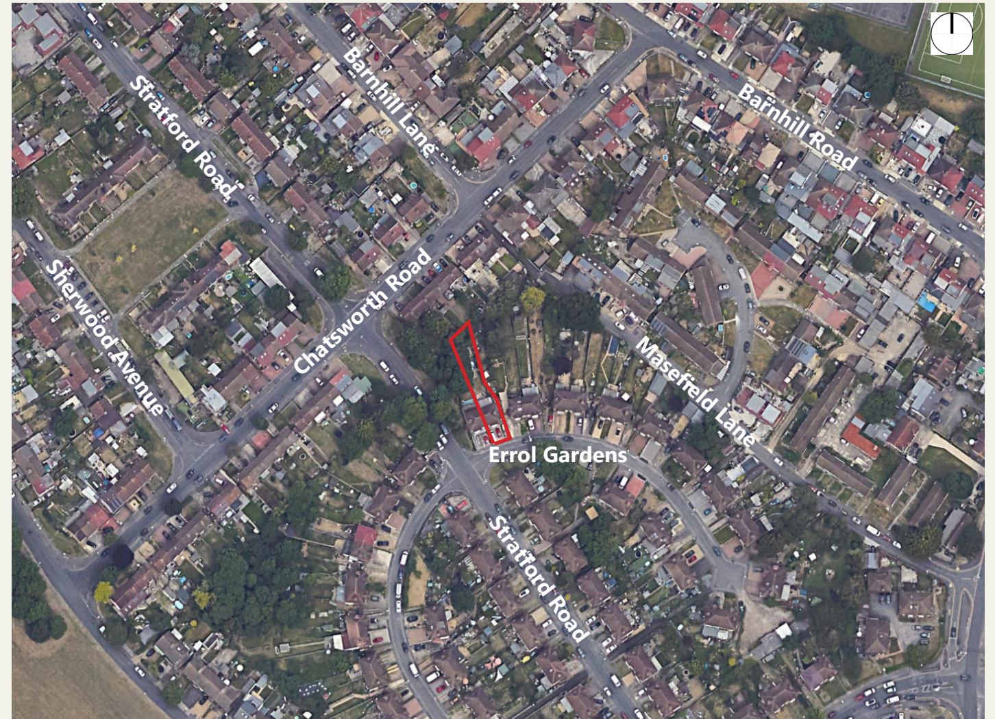
Fig. 01 Aerial view of 3 Errol Gardens, showing indicative boundary (highlighted in red)
