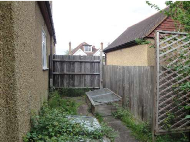
View from side of property (sub station).
