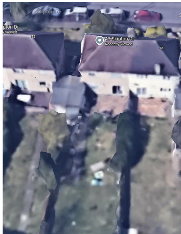
REAR AERIAL VIEW
