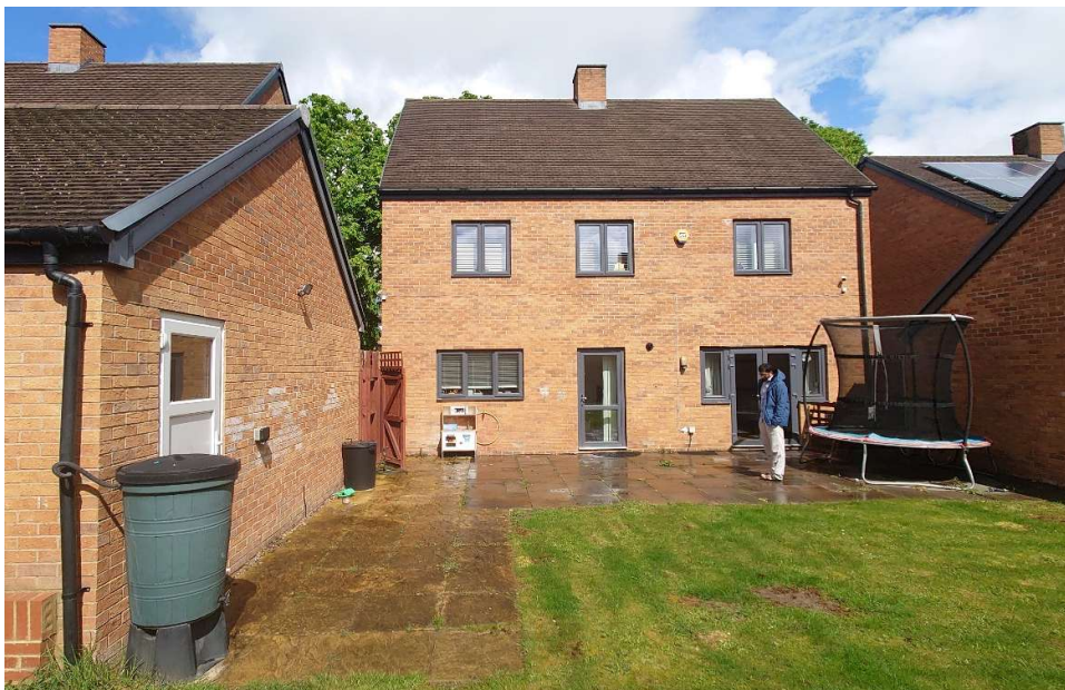
Image 2: Existing Rear Elevation of the Property
