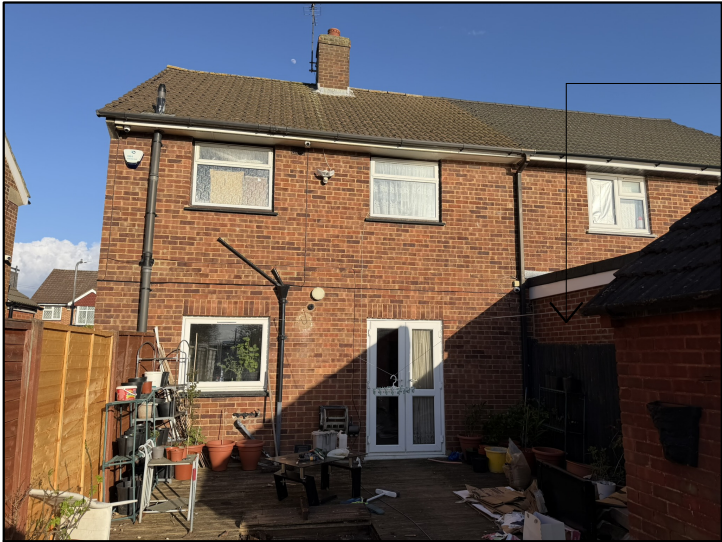
No 28 3M Rear Extension
