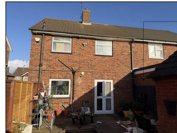
No 28 3M Rear Extension
