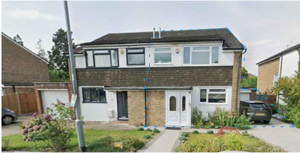
15 Foxfield Close Front Facade 1
