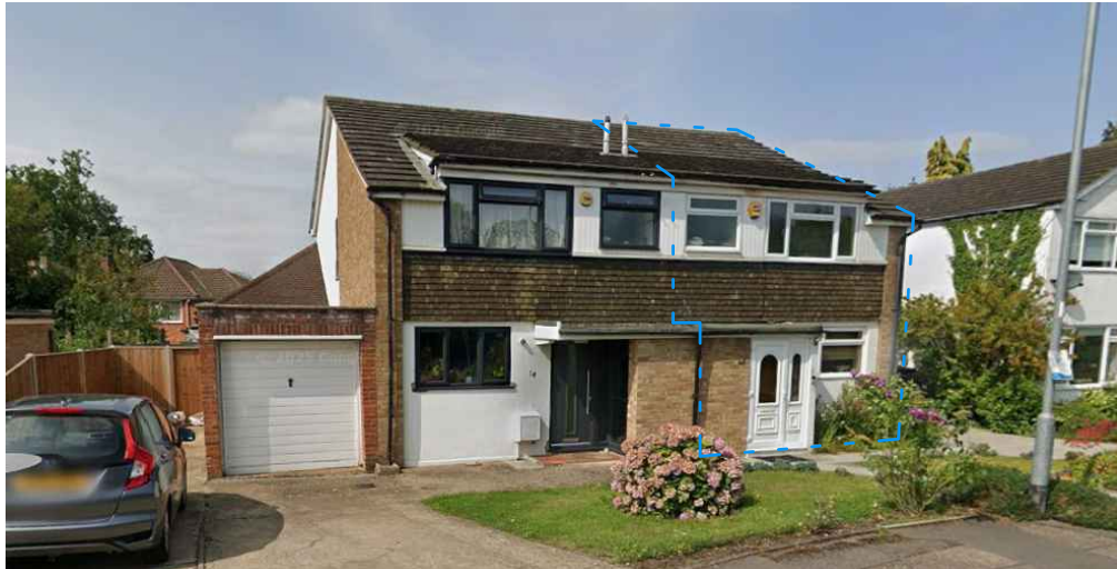
15 Foxfield Close Front Facade 3
