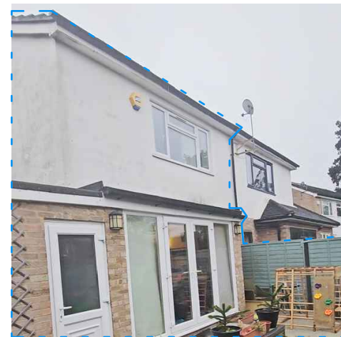
15 Foxfield Close Rear Facade 3
