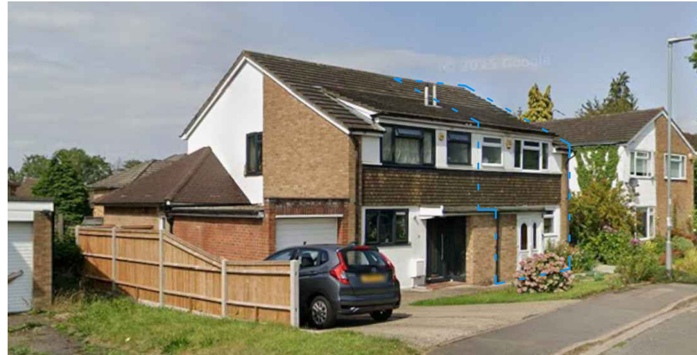
15 Foxfield Close Front Facade 4
