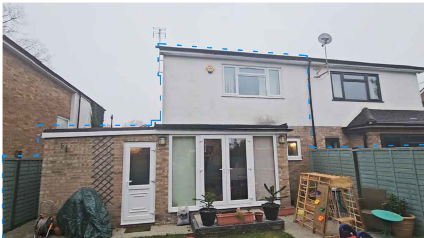
15 Foxfield Close Rear Facade 1
