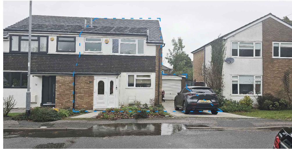
15 Foxfield Close Front Facade 2
