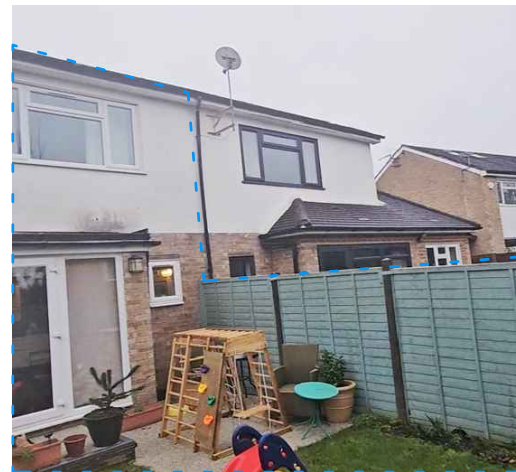
15 Foxfield Close Rear Facade 2
