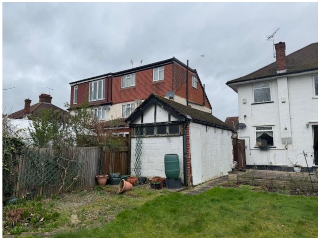
Photograph 08 – Rear view towards No. 100
