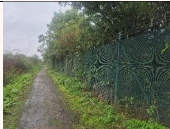
Photograph 100: Section 4: access track adjacent to STW
