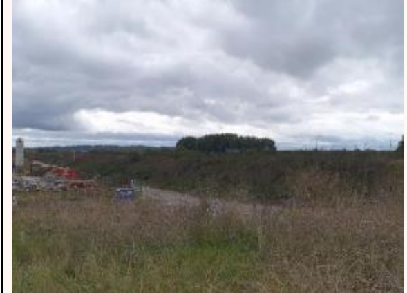
Photograph 41: Section 2: vegetated bund and quarry viewed from safe point
