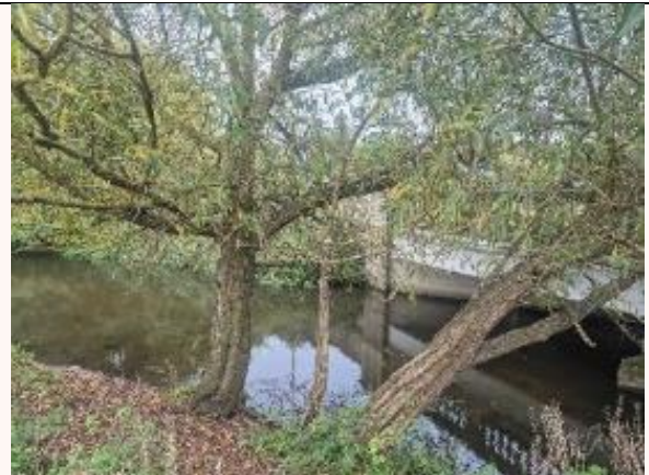
Photograph 90: Section 4: Colne Brook flowing under A4
